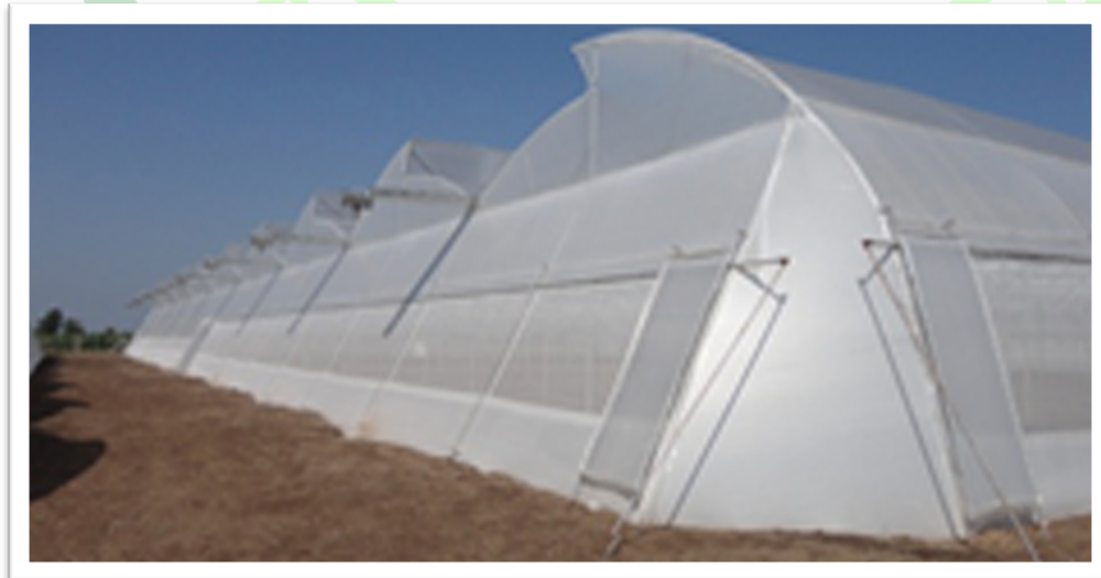
Naturally Ventilated Polyhouse
